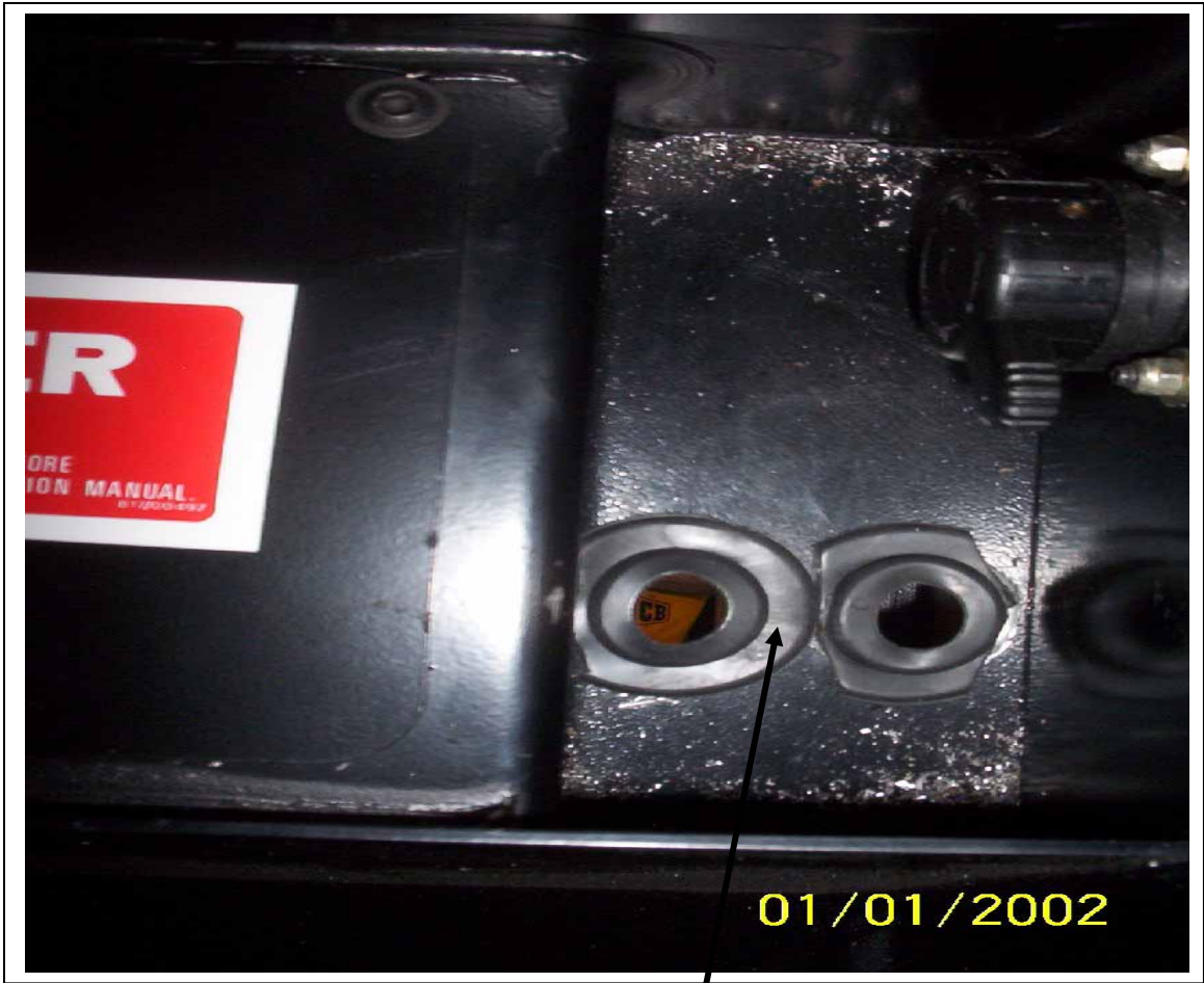
Grommets installed on 1 1/4" holes.
